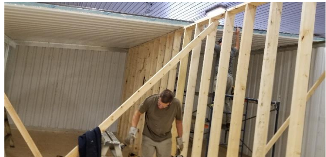
Figure 41: Temporary Support Wall with a mono pitch roof
