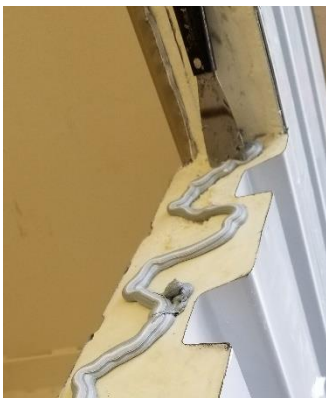
Figure 73: Serpentine bead of liquid flashing
