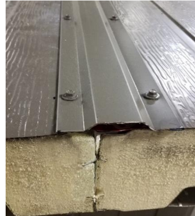
Figure 70: Roof Seam Cap installed with stitch screws spaced 16" apart
