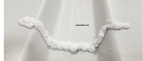
Figure 43: Foam Closures 1/2" sealant bead
