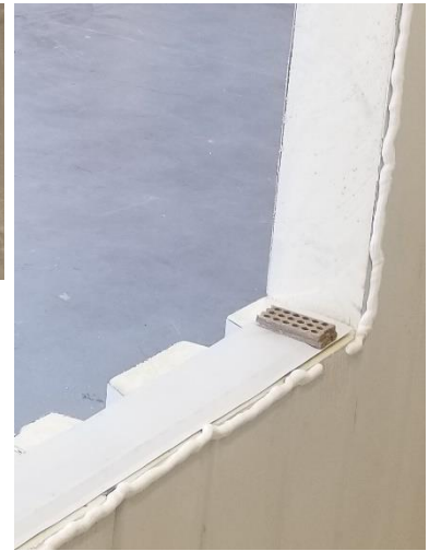
Figure 77: Sealant bead with drain gap
