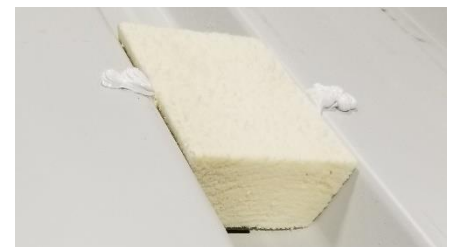
Figure 44: Installed Foam Closures
