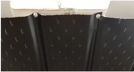
Figure 89: Fastening the Soffit
