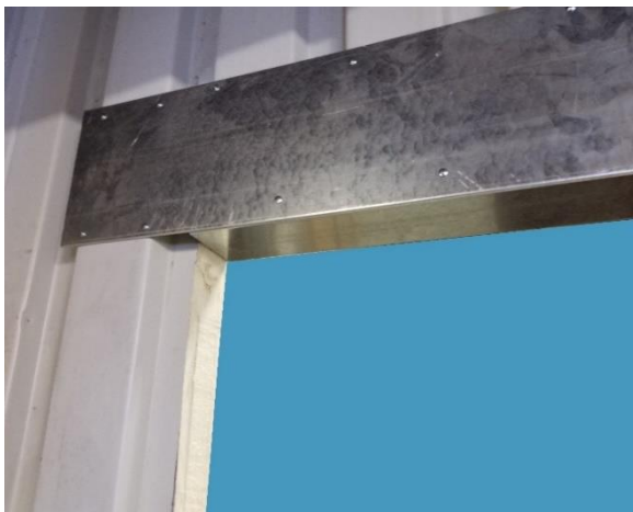
Figure 71: Header angle installed in window rough opening
