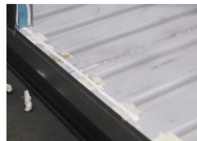
Figure 26: 1” sealant bead on floor
