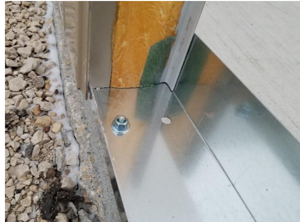
Figure 5: An installed base channel
