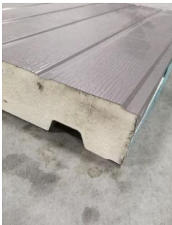
Figure 6: Tenon Side
