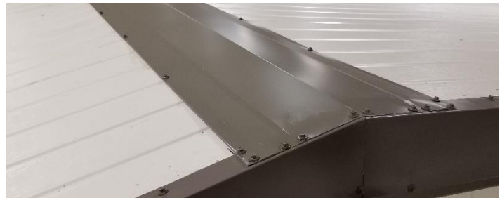
Figure 96: Colored stitch screws fastening the Ridge Cap
