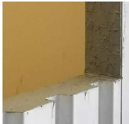
Figure 74: Properly spread liquid flashing
