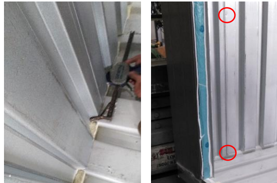
Figure 27: Panel Clamping Figure 28: Screw Placement
