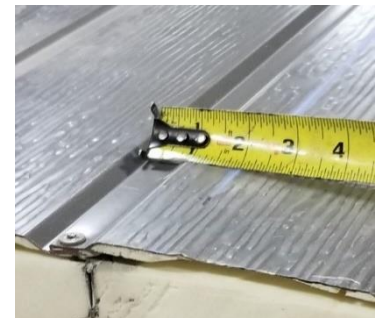
Figure 64: Snap a chalk line 2" from the seam.
