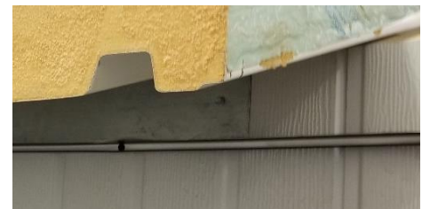
Figure 86: Installing Soffit J-Channel
