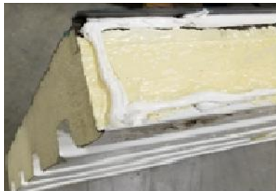
Figure 49A: Air barrier at the peak end, down the side and across the lower lip of the roof panel
