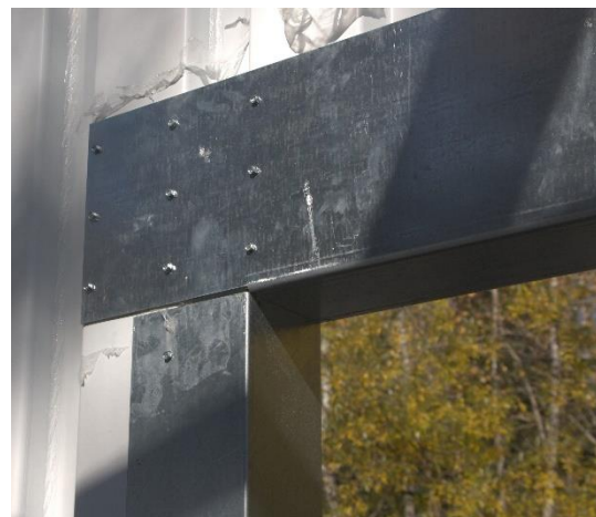
Figure 72: Header installed in garage door opening
