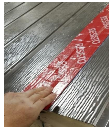
Figure 67: Applying the barrier
