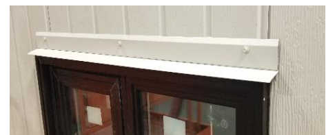
Figure 82: Completed window cap
