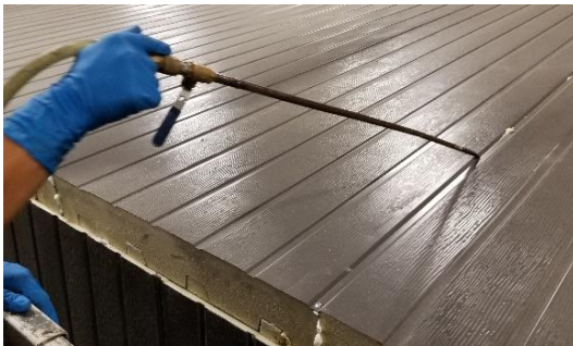
Figure 61: Removing debris from the roof panel joint
