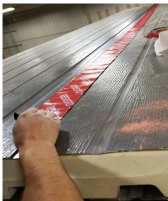
Figure 66: Aligning the barrier with the chalk line
