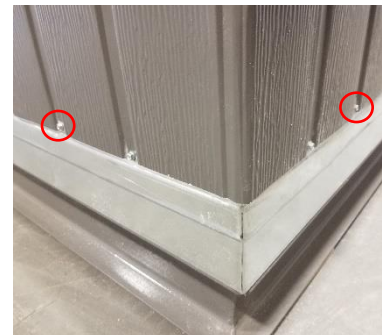
Figure 25: First Corner Installation
