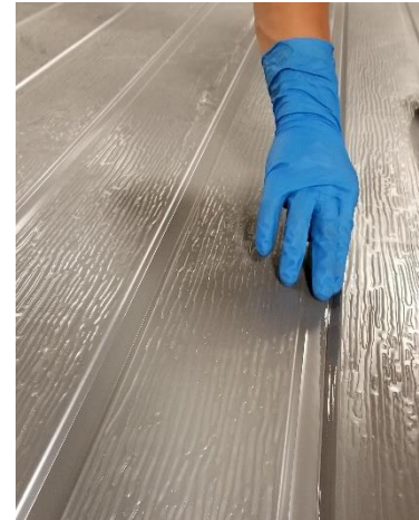
Figure 63: Working the silicone into the joint
