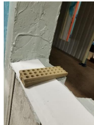
Figure 75: Shim support flashing and shims
