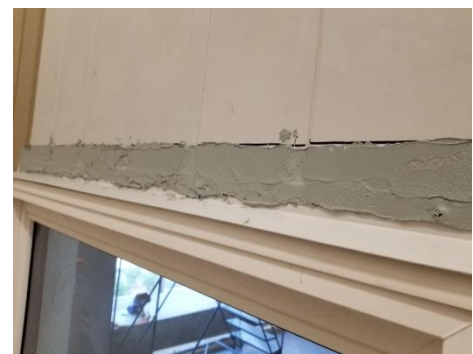
Figure 81: Liquid flashing spread to manufacturers thickness specifications
