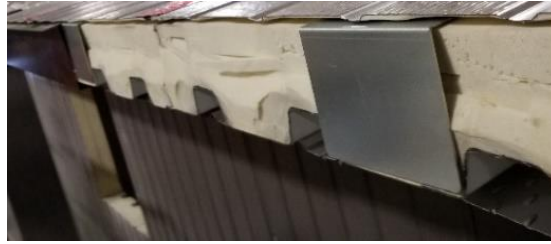
Figure 90: Eavestrough backing in the middle of each panel
