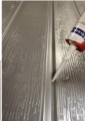
Figure 62: Applying silicone to the joint
