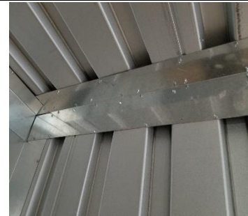
Figure 34: Floor to Wall Angle
