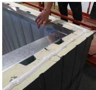
Figure 45: 1" polyurethane sealant bead 1 1/2" in from outside
