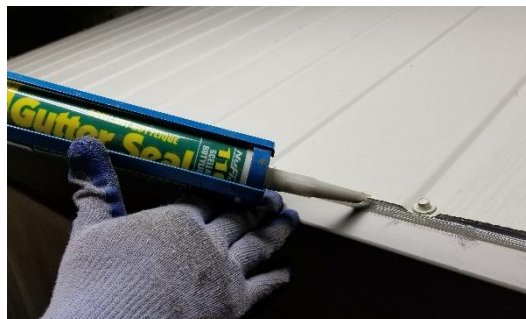
Figure 59: Sealing the roof eave kerf
