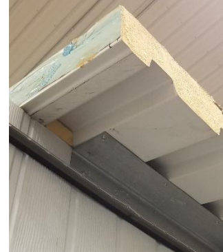
Figure 37: Exterior wall to roof angle with J-Channel for soffit installed
